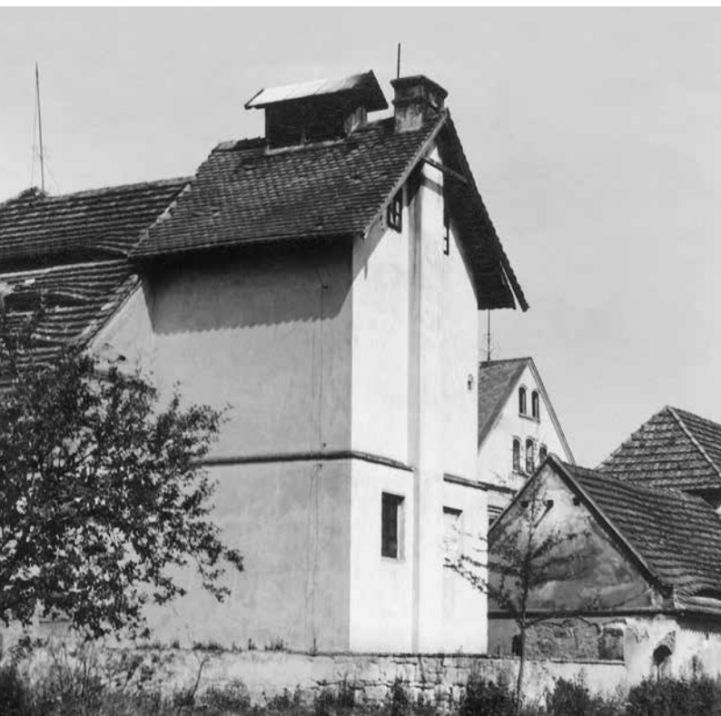
Rural hop drying kiln with an evaporator on the roof, attached to the barn, Saaz hop growing region, early 20 th century
