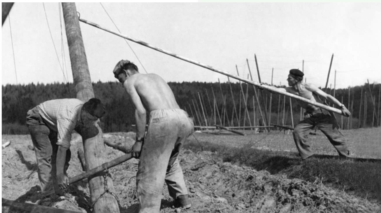
Erection of a frame column during the construction of a hop trellis, Saaz hop growing region, mid-20 th century
