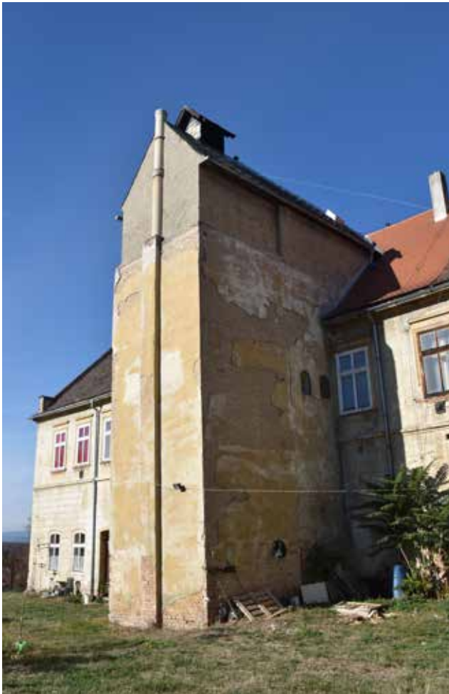
Chamber hop drying kiln with an evaporator on the roof, house No. 30, Dvořákova St., Žatec, 2016
